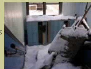
South stairs: Outside Kerr's room
